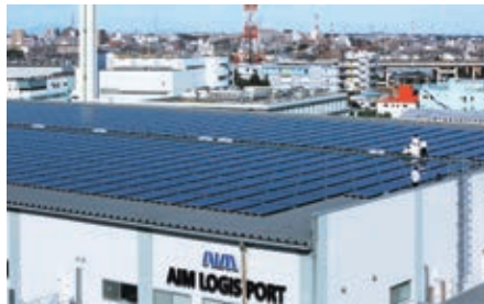
Solar power generation facilities were installed at AIM Logisport in 2014. Annually, these facilities generate enough electricity to power 100 households.
